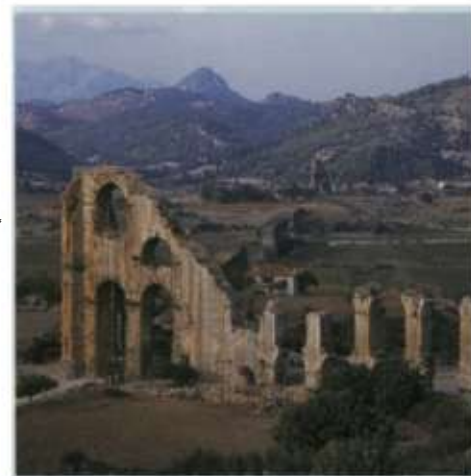
▲ Roman aqueduct at Aspendos, western Turkey, part of the Roman and later Byzantine Empires. The aqueduct brought water from the surrounding mountains to the city on the hill. The Romans were skilled engineers and built on a monumental scale.
